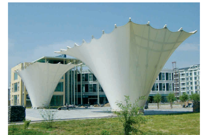
Example of asymmetrical curvature shapes with symmetrical primary structure, only generable by using VARIO-STRETCH fabric, properly compensated.
